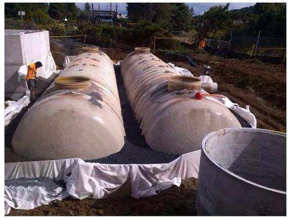
Figure 1: Tank installations during backfilling operations
