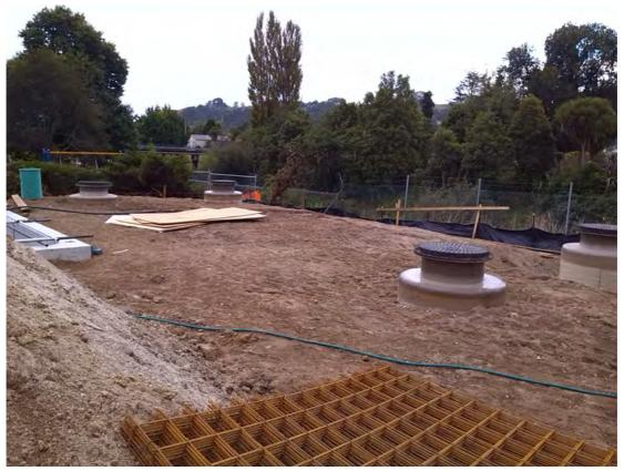
Figure 2: Tanks after backfilling operations
