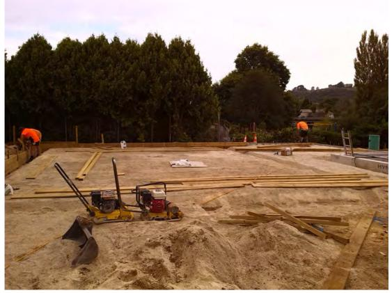
Figure 3: Building floor slab preparation
